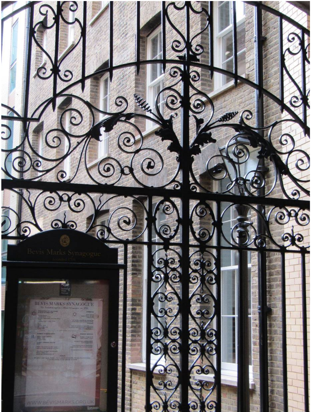
Fig. 8: Rear elevation of Nos. 11-12 Bury Street, seen through courtyard entrance gates
