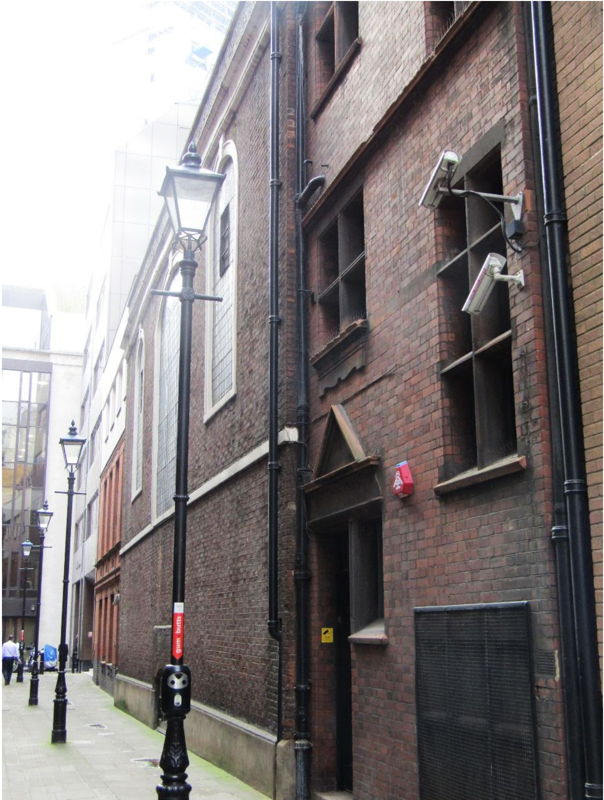
Fig. 5: Beadle's House (foreground) with neighbouring E elevation of Synagogue, Heneage Lane
